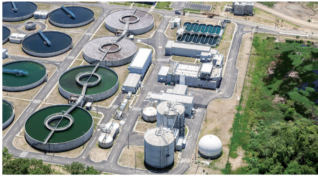
Inaugurated by Panamanian President Ricardo Martinelli in August 2013, the Juan Dian Wastewater Treatment Plant is the centerpiece of the Panama City and Bay Sanitation Program. Designed, built, and operated by Nippon Koei LAC, it uses activated sludge technology and has facilities to convert wastewater sludge to electrical energy.
