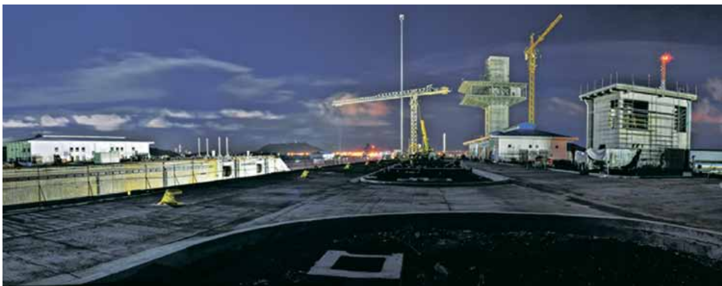
With the inauguration of the Third Set of Locks of the Panama Canal, the world-famous waterway has allowed the passage of larger ships and as a result, maintained its advantage over its competitors. As the country continues building more infrastructure, Japanese construction and engineering firms remain major players in this nation-building endeavor.
