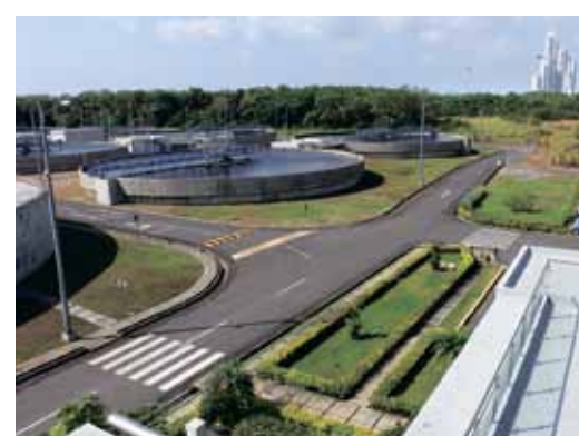
Through the Juan Diaz Wastewater Treatment Plant, Nippon Koei LAC helped Panama City, one of the world's fastest-growing cities, meet its infrastructure needs.
