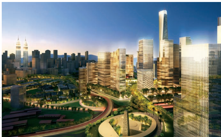
Tun Razak Exchange, the 70-acre international financial district in Kuala Lumpur, begins construction in 2013.
