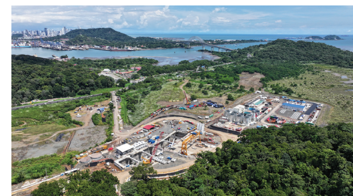
Panama's Metro Line 3 will pass beneath the Panama Canal.
